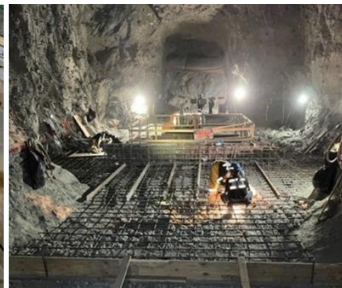
Grizzly installation and truck ore loading pocket foundation pours
